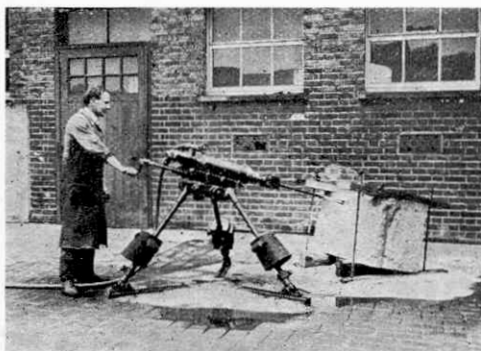
A Rock Drill driven by a 2 h.p. engine, and invented in 1914
