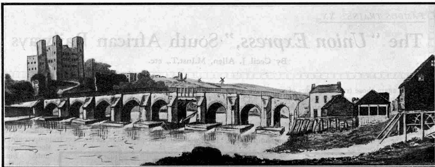
The bridge across the River Medway at Rochester, with the old tide mill on the right. The water required to work the mill was stored at high tide in large ponds, where it was retained as the level in the river fell until the head of water was sufficient for successful working. Two windmills are to be seen in the background
