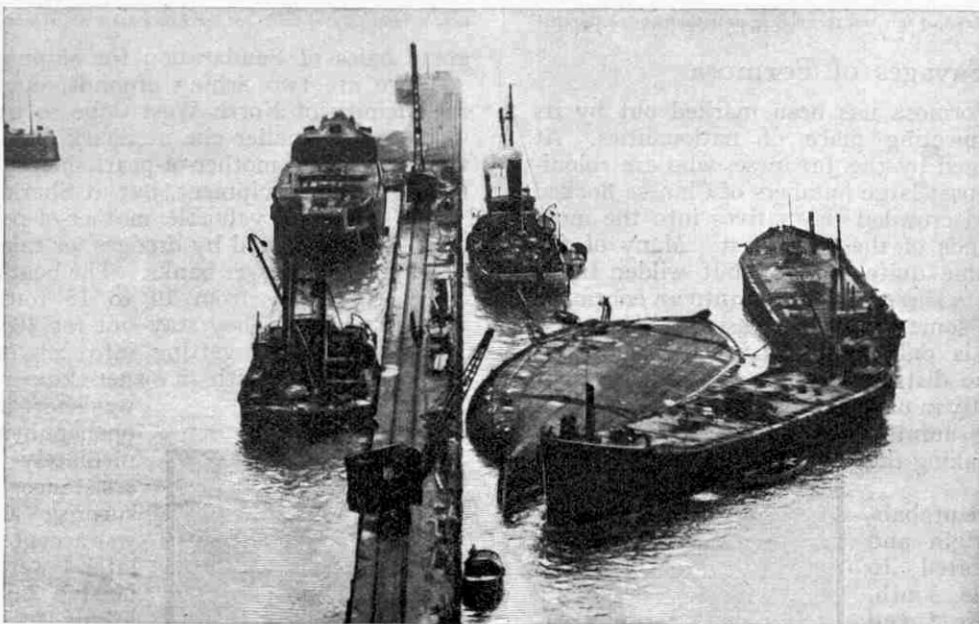
H.M.S. "Glatton," the overturned monitor, surrounded by salvage vessels. She is being coaxed alongside the eastern arm of the submarine harbour at Dover. The vessel was salvaged by the Harbour Master at Dover after many salvage firms had refused to undertake the difficult task. (From "Perilous Days" reviewed on the previous page)
