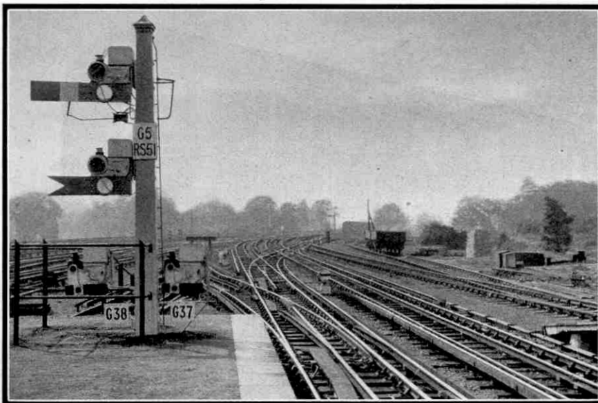
Permanent Way at Wembley Park showing the Westinghouse Signalling equipment
