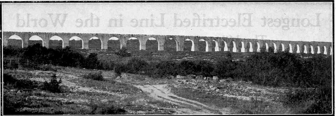
Engineering of 2,000 years ago ! A Roman aqueduct still standing in France as evidence of the skill of Roman engineers.
