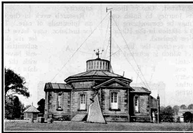
A closer view of the Meteorological Pavilion. This includes a wireless room and has magnetic chambers underground.
