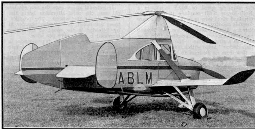
Another view of the cabin type of Cierva "Autogiro" shown opposite. This machine is fitted with a D.H. "Gipsy" Mark III inverted engine and has a cruising speed of 100 m.p.h. The upper illustration shows pilots of the U.S. Army Air Corps equipped for work at an altitude of five miles. The men breathe by the aid of oxygen apparatus and communication is maintained by wireless. Official photograph, U.S. Army Air Corps.
