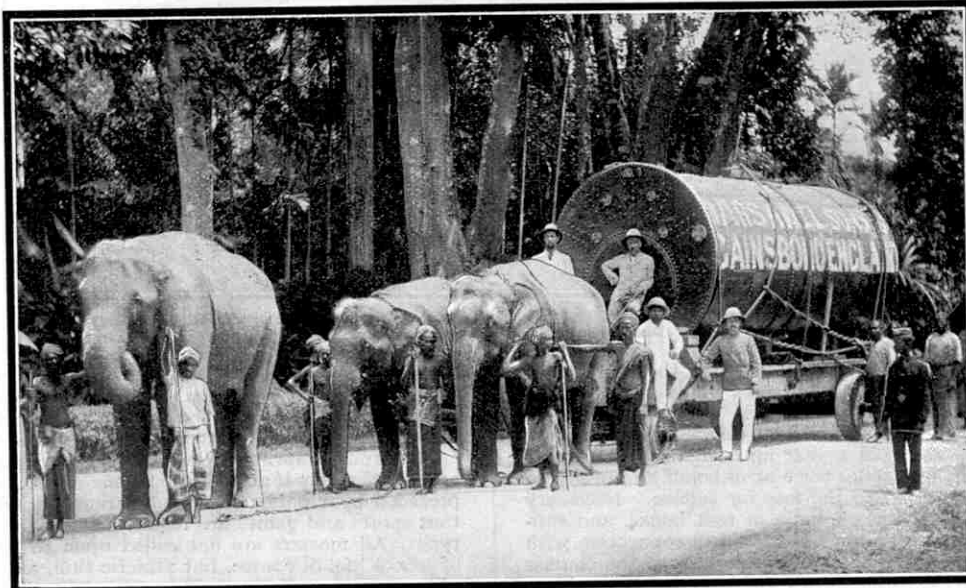
Transport methods in Ceylon. Elephants hauling a boiler that is to be installed on a tea estate. For this illustration we are indebted to Marshall, Sons & Company Ltd., Gainsborough.
