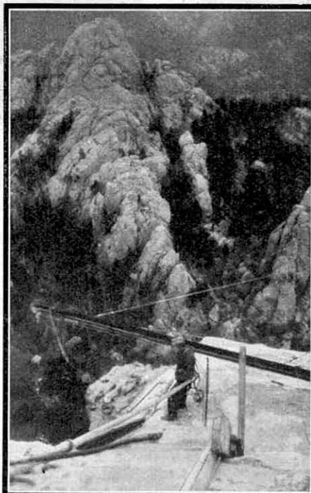
The "Steel Monkey"—a man who travels about the cliff in harness—delivering necessities to the men at work.
