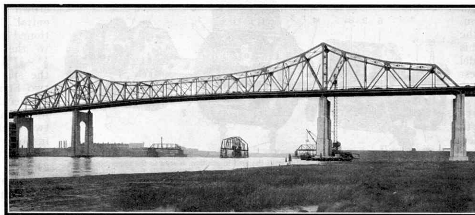
A fine view of Goethals Bridge, which spans the "Arthur Kill" Channel between Elizabeth, N.Y., and Howland Hook, Staten Island, a distance of 600 feet.
