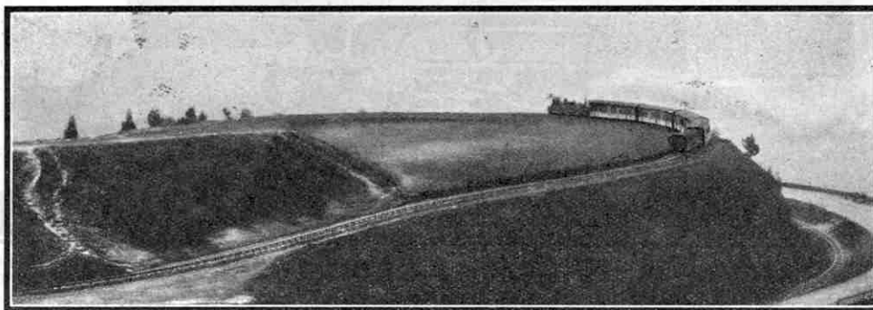
The Batasia Loop on the Darjeeling-Himalayan Railway. This loop is the last of a series by which the railway obtains an easy ascent over the steepest sections of the route.
