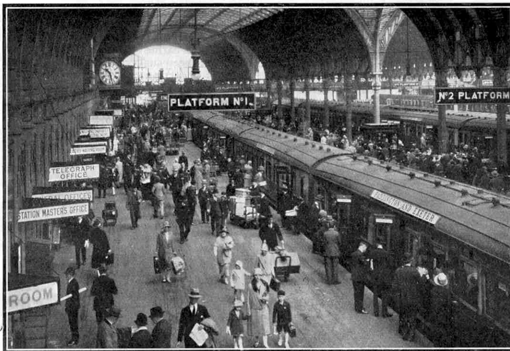
A busy scene on No. 1 Platform at Paddington immediately before the departure of the "Cornish Riviera Express." Many famous G.W.R. expresses are despatched from this long platform.
