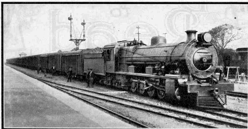
A train of 21 special grain trucks on the South African Railways conveying a bulk consignment of maize. Photograph by courtesy of South African Railways and Harbours.
