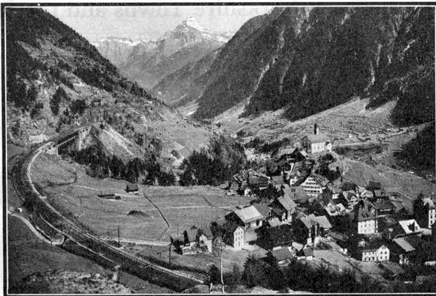
A picturesque view on the St. Gotthard line near Wassen. This village is passed three times at different levels by the railway on the ascent to the St. Gotthard Tunnel.
