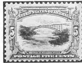
An under-arch bridge at Niagara Falls. This type of bridge is rarely found in engineering to-day.
