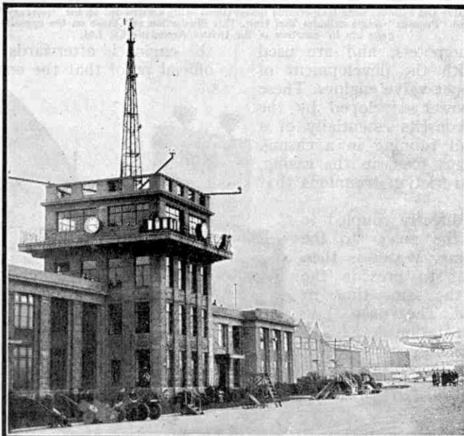
The Control Tower at Croydon Airport. Photograph by courtesy of "The Aeroplane."
