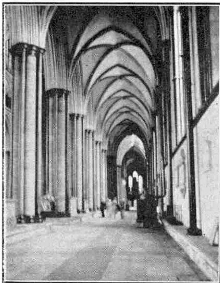
The decorated roof of Salisbury Cathedral.
