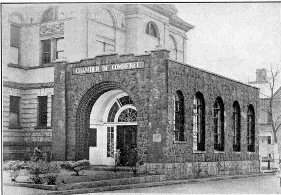
A building constructed of coal. The Chamber of Commerce building at Williamson, West Virginia, in the United States. Photograph by courtesy of the "Norfolk and Western Magazine."
