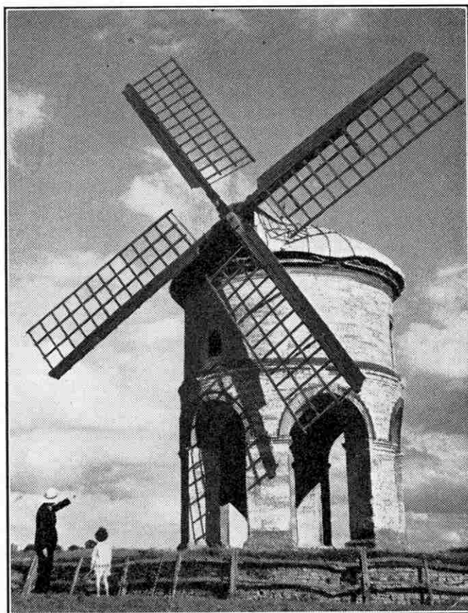
Chesterton Mill, Warwickshire. Photograph by C. H. Eaton, Hall Green, Birmingham.
