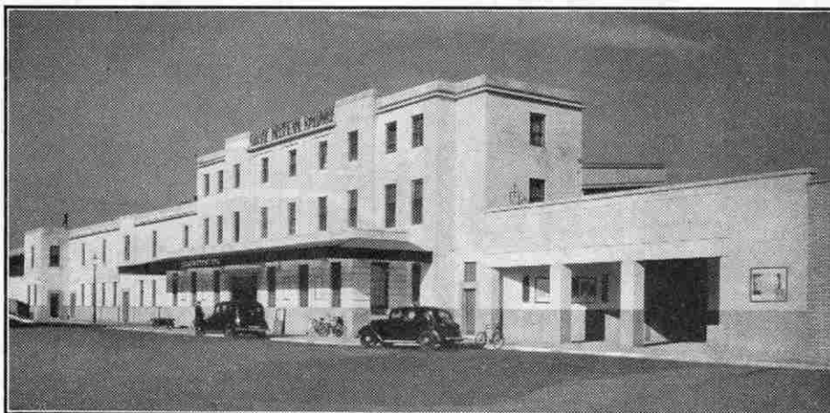
The imposing frontage of the new G.W.R. station at Leamington Spa. Photograph by courtesy of the G.W.R.
