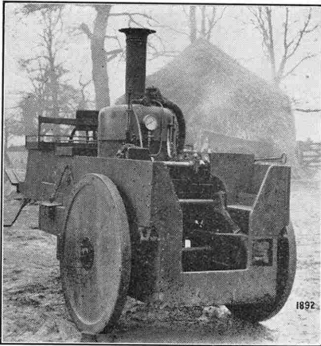
The Carriage seen from the rear.
