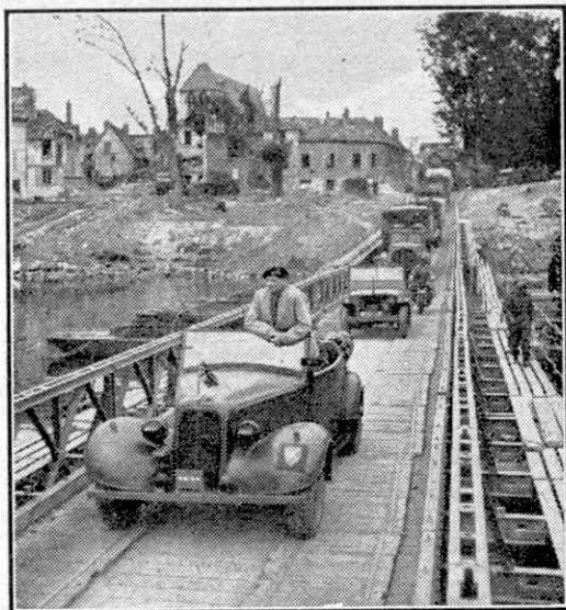
Field Marshal Montgomery crossing a Bailey Bridge over the Seine at Vernon. The bridge surface is laid with the Sommerfeld portable track. The illustrations to this article are British Official Photographs, Crown Copyright Reserved.
