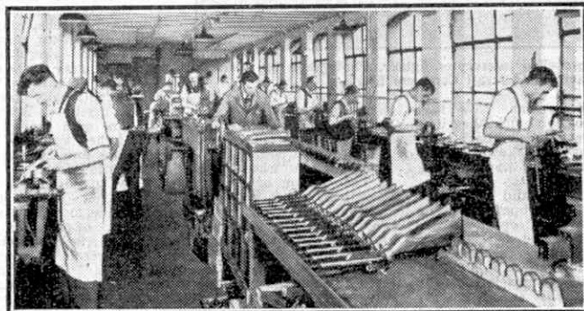
Making Webley Air Pistols and Air Rifles; the assembling department. Our photographs are reproduced by courtesy of Webley and Scott Ltd., Birmingham.
