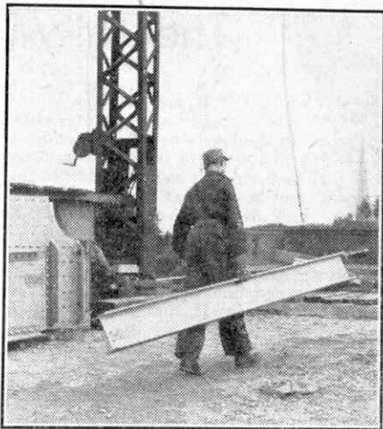
One man can easily pick up a large metal girder, and walk briskly away with it, if the metal is an aluminium alloy. Photograph by courtesy of the Aluminum Company of Canada Ltd.
