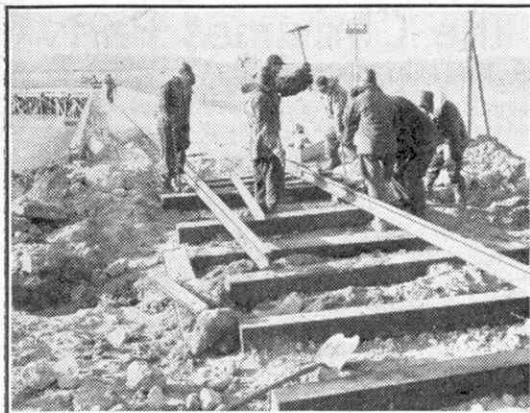
Laying the track of the Labrador railway northward out of Seven Islands towards Burnt Creek, centre of the iron ore fields of Labrador.
