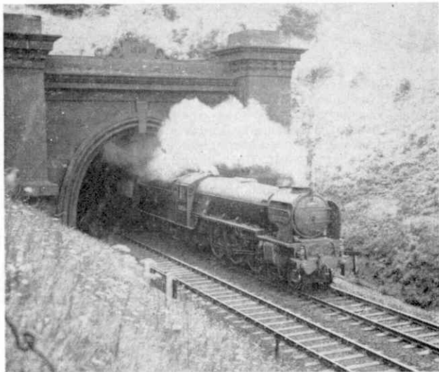
"The Heart of Midlothian" headed by No. 60154 "Bon Accord" leaving the north end of Welwyn North Tunnel. Photograph by S. Redhead.
