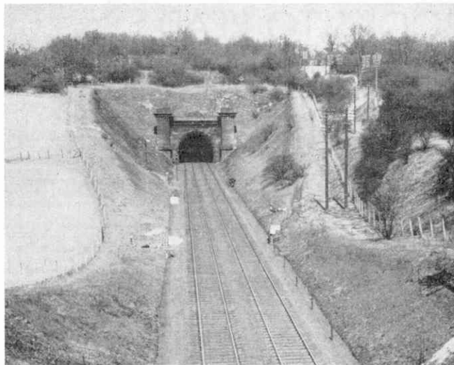
South end of North Welwyn Tunnel, seen from the north end of the South Tunnel. British Railways Photograph.
