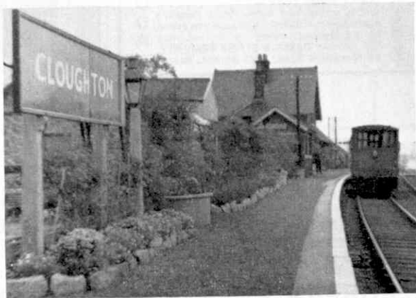
Cloughton Station, on the line between Scarborough and Whitby. Photograph by H. D. Walkland, Northallerton.
