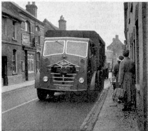
Here is a section of A5, claimed to be the busiest commercial highway in Europe, passing through the village of Markyate, Herts., where it is only 16 ft. wide and the footpaths are correspondingly narrow. Photograph, "Picture Post" Library.
