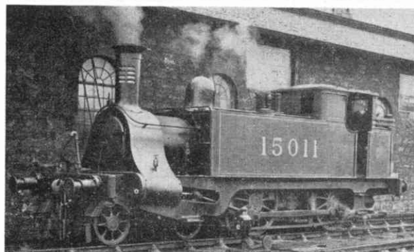
The style of earlier Highland locomotive construction is well shown by this quaint little 4-4-0T, L.M.S. No. 15011. It was built in 1878.
