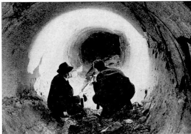
A peep into the pilot tunnel which already exists under part of the English Channel. Photograph by courtesy of the Society of Motor Manufacturers and Traders.
