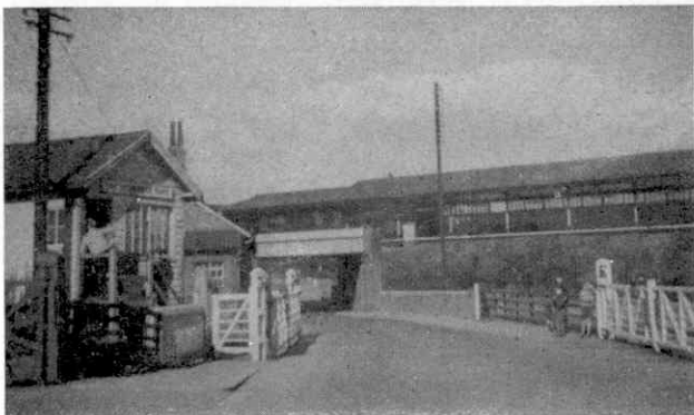
Over the bridge seen down the road the famous East Coast Route expresses run through Northallerton Station, which is built partly on the bridge.
