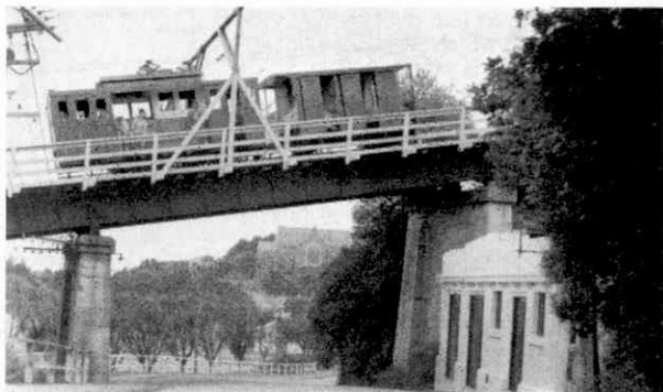
Another section of the 2,574 ft. Wellington cable railway, the gradient of which is about 1 in 5.
