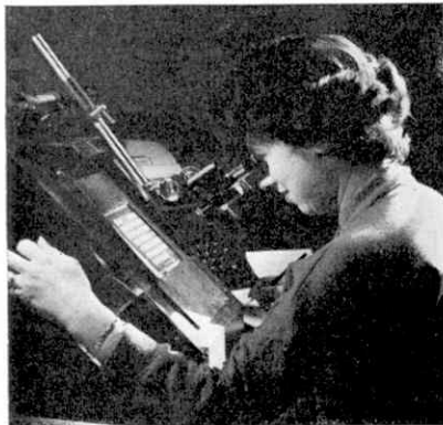
A member of Bristol Siddeley's Flight Test Department is seen examining, on a film reader, the recordings taken from an Automatic Observer Panel.
