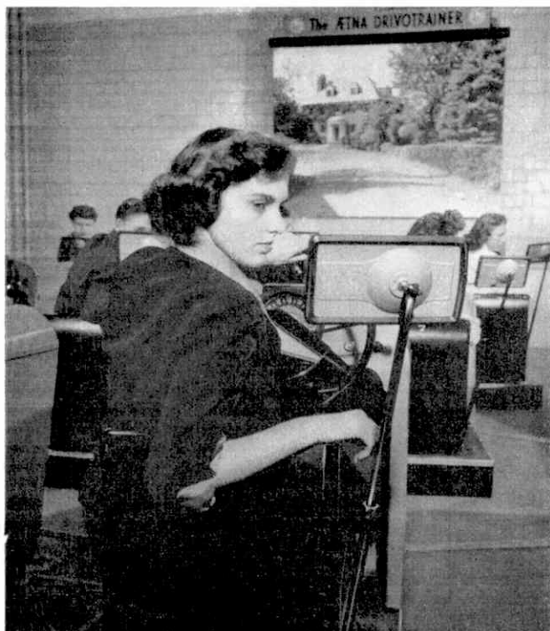
Left: Driving backwards in the stationary cars used with the Drivotrainer. The student looks into the mirror to see the driveway shown on the screen in the same way as if looking through the rear window of an actual car. Right: The automatic scoring system permits the instructor to follow the performance of each pupil simultaneously at a central recording unit. The actions of each student driver are printed on the score sheet, which also serves as a permanent record of progress. These pictures are reproduced by courtesy of Aetna Life Affiliated Companies, Conn.
