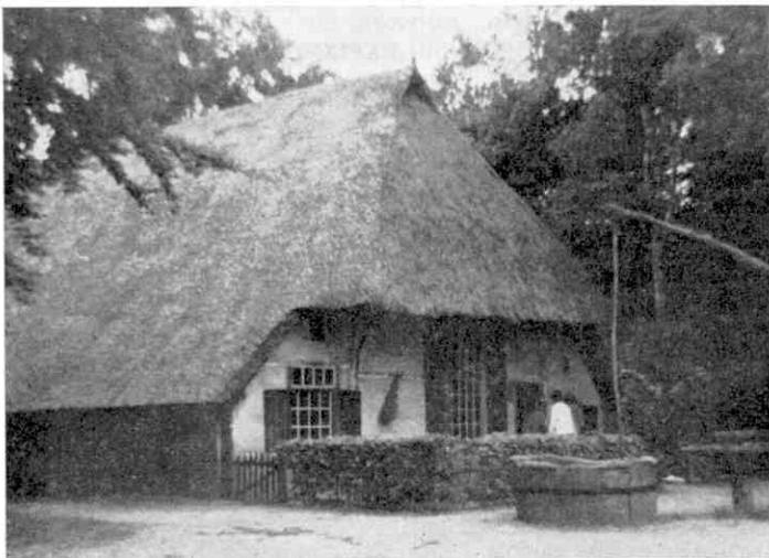
A "loshoes" farmhouse from the Achterhoek region in which the threshing floor, the stalls for livestock and the living accommodation all form a single unit.
