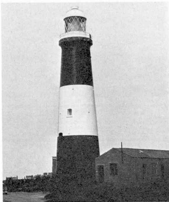
Above: There's nothing temporary about a Lighthouse. Types such as the Eddystone one are immensely strong and built to last for many years. Opposite: All Penzance depot buoys are overhauled prior to re-siting.
