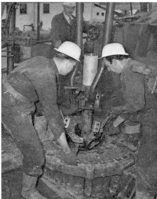
Below: Two men are shown lowering a drill pipe into position. A B.P. photograph.
