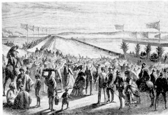
Sightseers flocked to see the Canal being officially opened a century ago.
