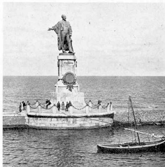
A statue of Ferdinand de Lesseps, the French engineer who conceived the Suez Canal, and who supervised the construction work, overlooks the entrance at Port Said.
