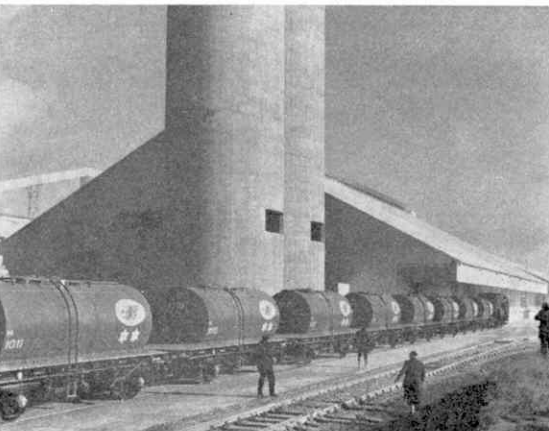
Below: Bulk carriers taking clay slurry by rail to home consumers.
