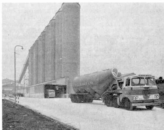
Above: Bulk tanker pressure loaded with powdered clay leaving storage silos.
