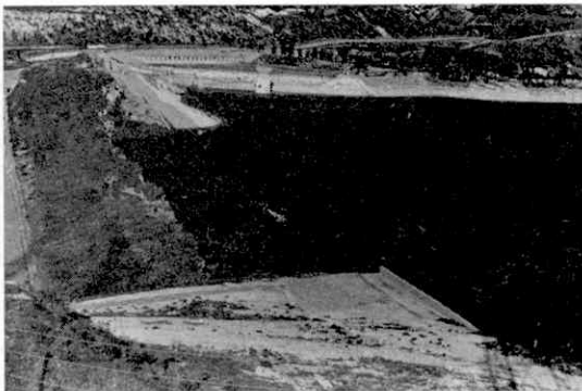
Below, a barely visible L.A. City Police Dept. Bell 47 'copter inspecting the section of the Van Norman Dam which collapsed in the recent earthquake (pic. by Los Angeles Times) and, bottom, $20,000,000 damage to the freeway interchange complex just outside Los Angeles. Note collapsed overpass sections.
