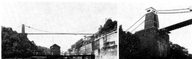
assembly bolted together. Sixteen such chains were used, in four sets of four. They were replaced by new ones of high tensile steel about 1940. The bridge deck was 30 feet wide with two 12 foot carriageways and a six foot footway in the centre, and was carried on suspension rods spaced at five foot intervals. These rods were one inch square in cross section and hung from the chain joints, which were staggered to suit this five foot interval.
