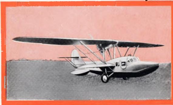
situated one in the bows and the other aft of the wings, and the pilots and navigator are accommodated in a small cabin in front of the wings. A Bristol "Pegasus" engine driving a pusher airscrew is mounted on a nacelle carried on struts between the wings.
